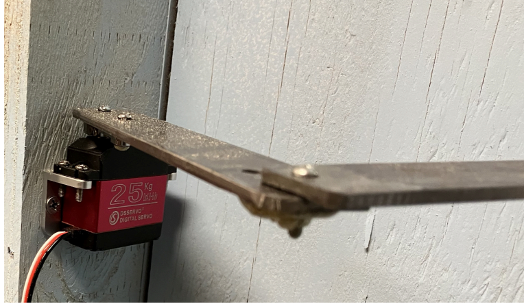
Fig. 4: Active Window Mechanism Servo Mounted on Window Frame
